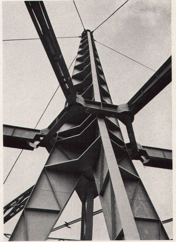
4 The girders before positioning of the roofing slabs 5 Main upright with the hexagonal suspension member for the main girder 6 The roof after completion of roofing slab fitment
