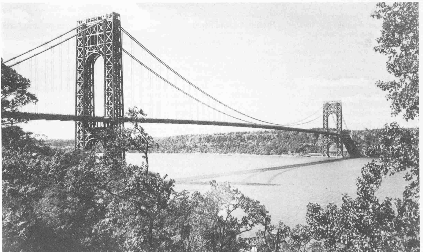
George Washington-Brücke in New York (1931)
