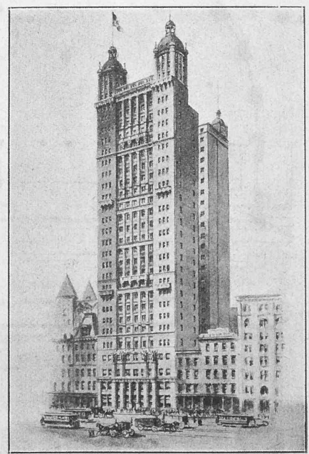
Abb. 17. New-York. — Park Row Office Building.
