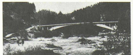
2051 Schwarzenburg 1932 Rossgrabenbrücke, Ing. Maillart Robert
