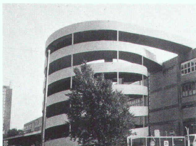
Rampe de parking Migros Herdern
