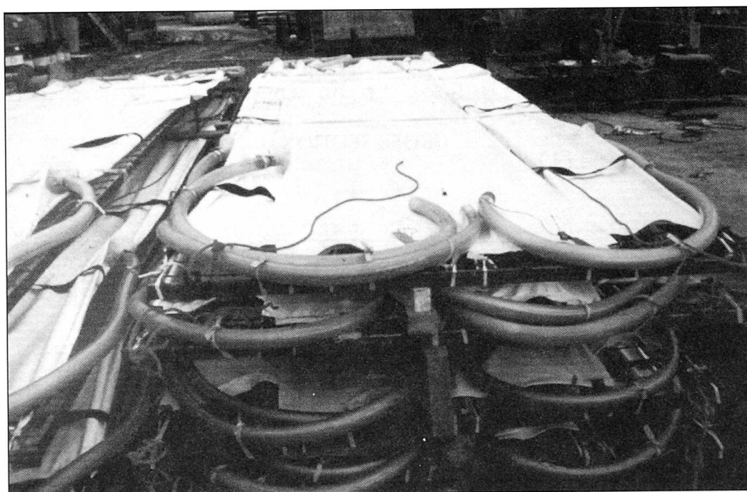
Fig. 5 Sacks before injection
