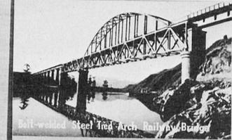
**Belt-welded Steel Truss Arch Railway Bridge**
