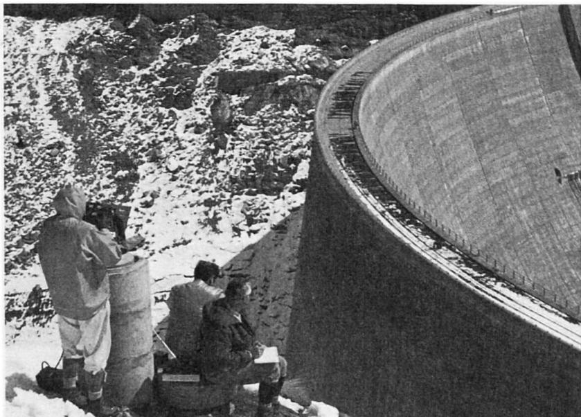
The Mekometer used for dam control measurements
