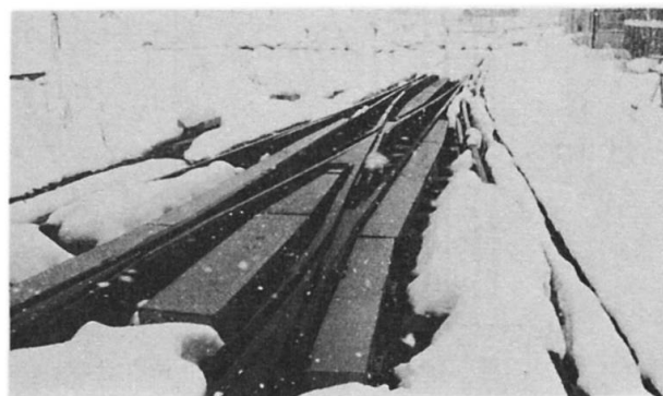
Photo 2 Snow melter for turnout
