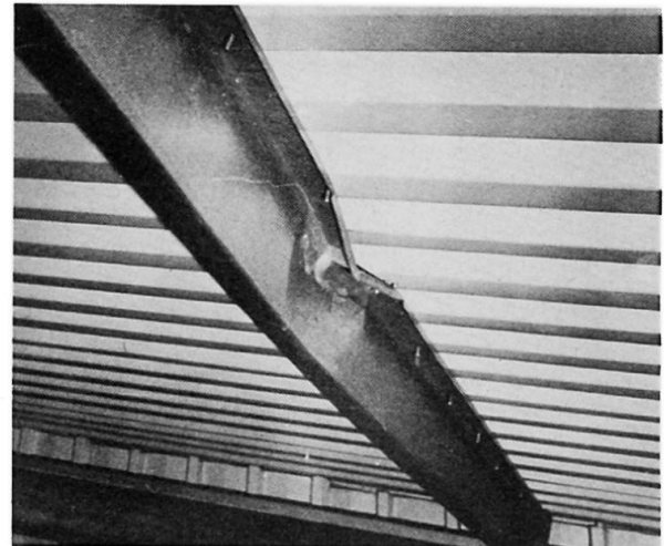
Fig.3 Buckled Z-purlin.
