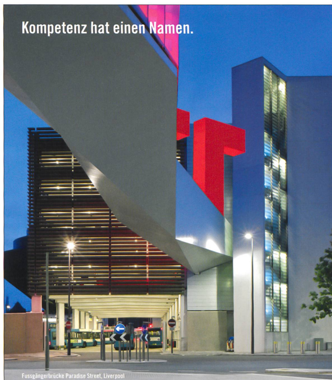
Fussgängerbrücke Paradise Street, Liverpool
