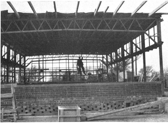
North Lancing School, Stahlskelett / Ossature métallique / Steel frame
