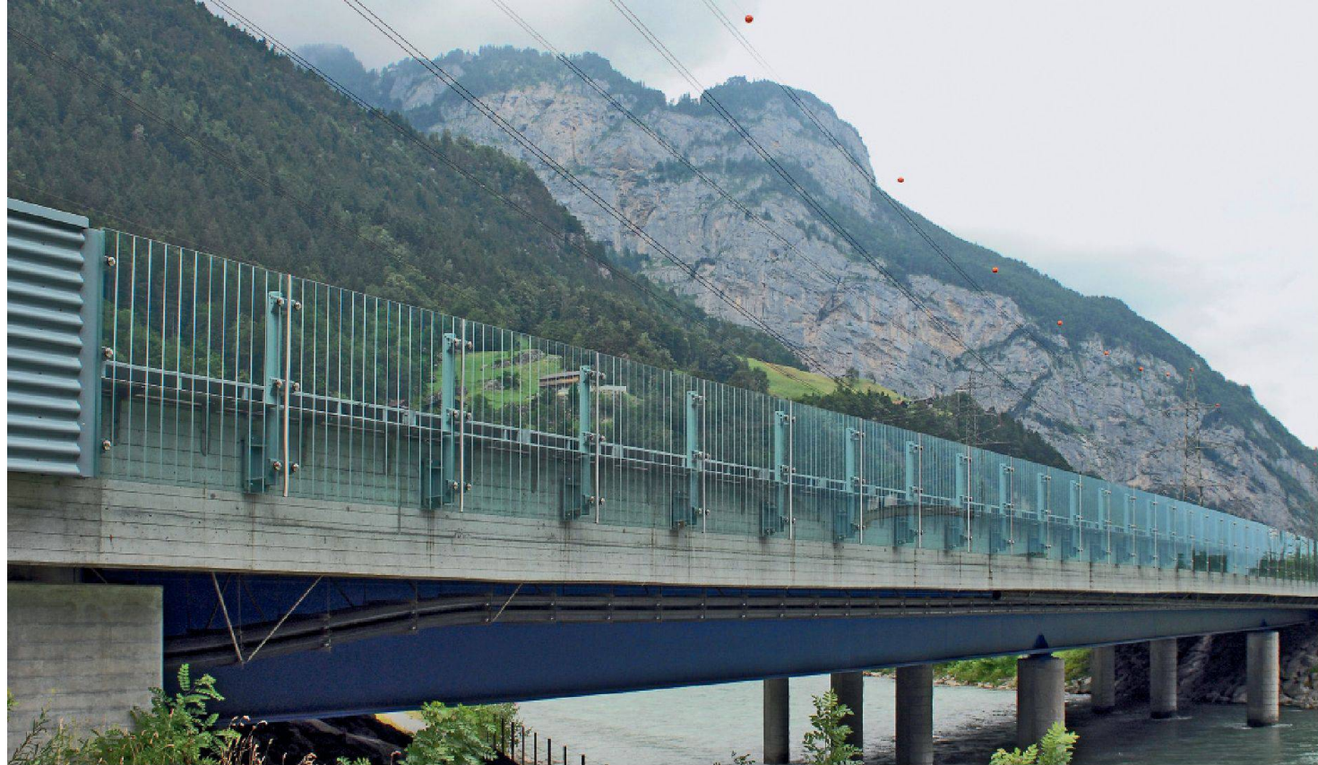
01 The new self-draining asphalt and noise barriers reduce noise pollution in the Reuss Valley (photo: Joe Müller)
