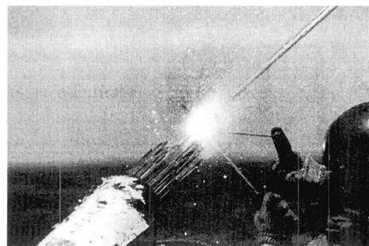
Fig. 4 Removal of existing cable by cutting of individual wires
