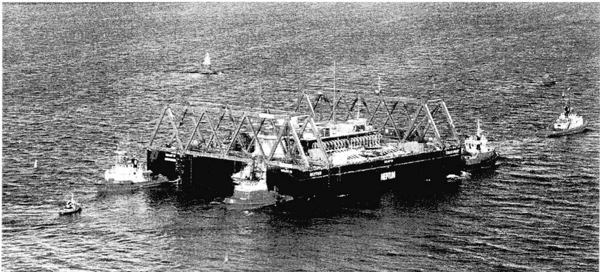
West Caisson during Towing
