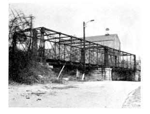
Fig.2. Bollman's Suspended & Trussed Bridge (1869) was relocated from a main line of the Baltimore & Ohio RR to service the mill at Savage, Maryland. It is the only known example of its type and facilitated the rapid expansion of early American railroads westward. Robert Vogel, Smithsonian Institution.
