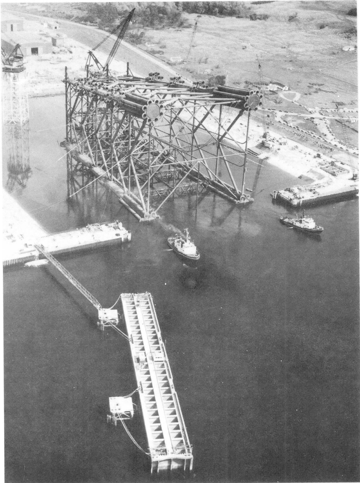
Fig 7 A self-floating petroleum production platform under tow from the construction dock of Brown and Root-Wimpey Highlands Fabricators Limited to the Ninian Field of the Chevron Consortium. The guides for the supporting tubular piles can be seen at each corner of the structure
