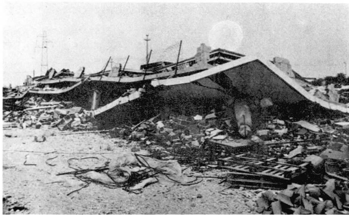
Figure 8: (after September 15th): Wreckage of the residential and business house near Artegna. The groundfloor of the building collapsed during the earthquake of September 11th. Through the impact, the undamaged living storeys also collapsed. The destroyed fixing points of the reinforced concrete columns in the groundfloor as well as the cracked brick walls of the staircase were not enough to carry the renewed strong earthquake stress. The experts had hoped, despite the doubts of the owner, to be able to repair the building.
