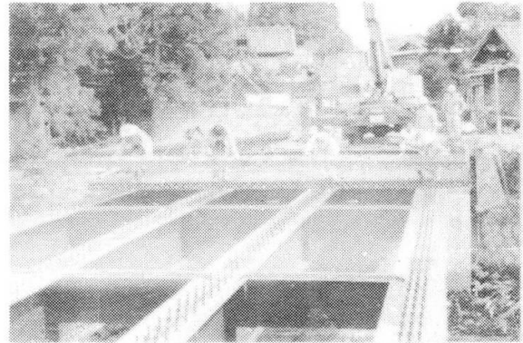
Fig. 12 Setting of I.B GRATE Floor
