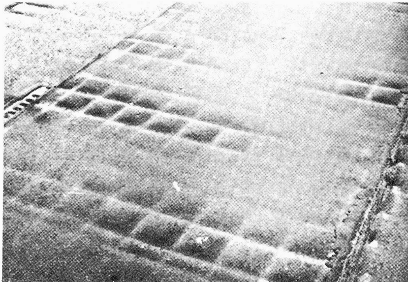
Figure 13: Steel mesh anchoring; plasterlike top surface
