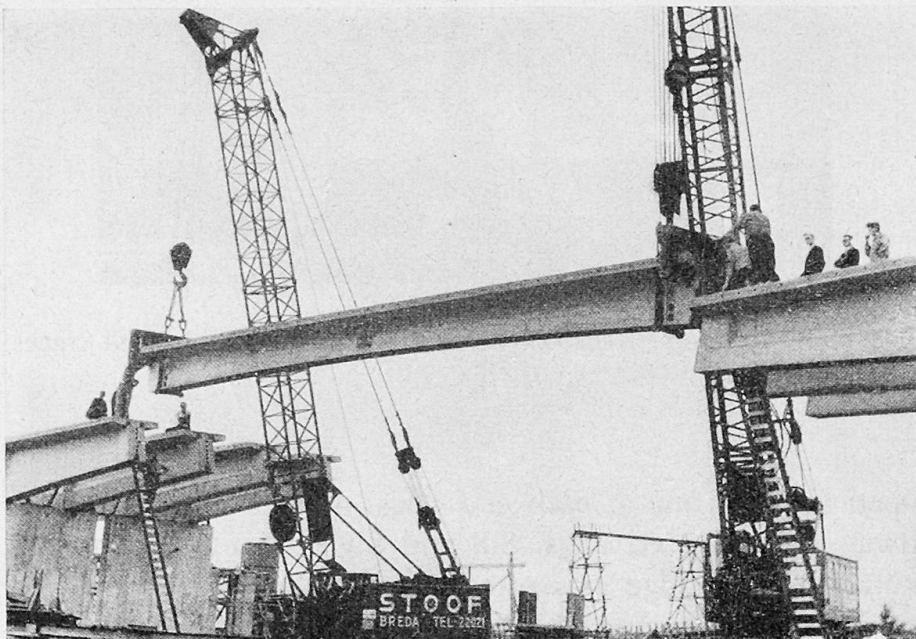
Fig. 4.5 - Handling a bridge element by two movable cranes.
