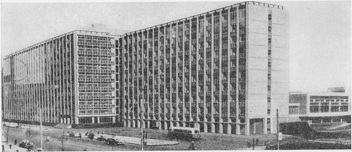
Fig. 6.2 - The finished building (tric-foto).
