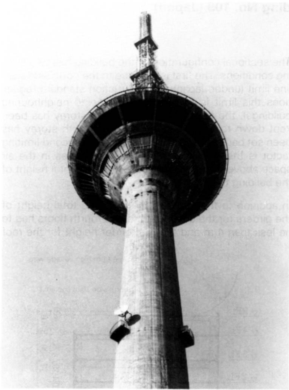
Fig. 2 Television tower view showing partly skypod floor and antenna
