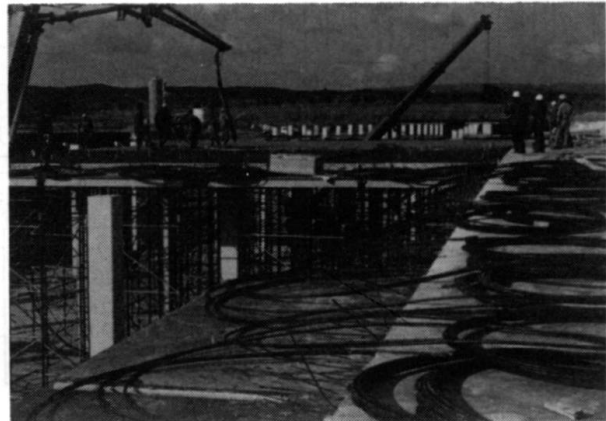
Fig. 6 One of the roofs during concreting of a segment
