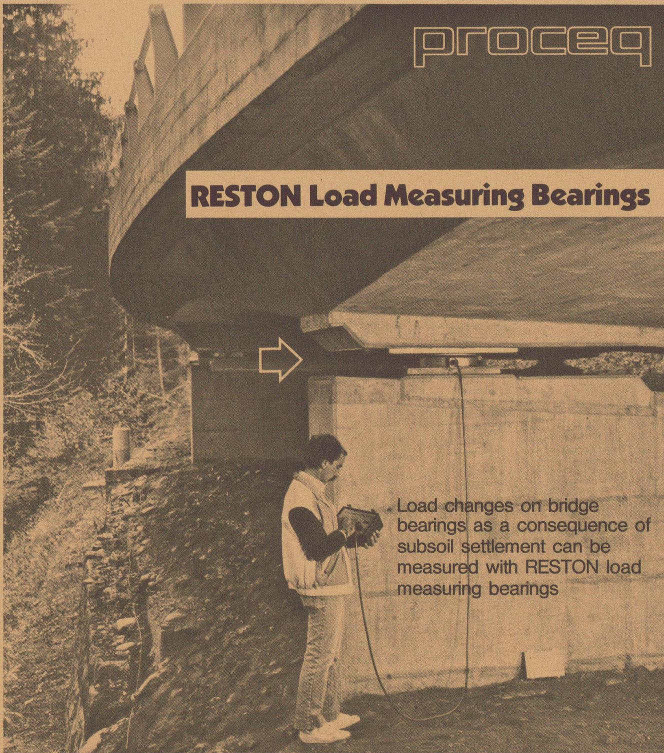
Load changes on bridge bearings as a consequence of subsoil settlement can be measured with RESTON load measuring bearings
