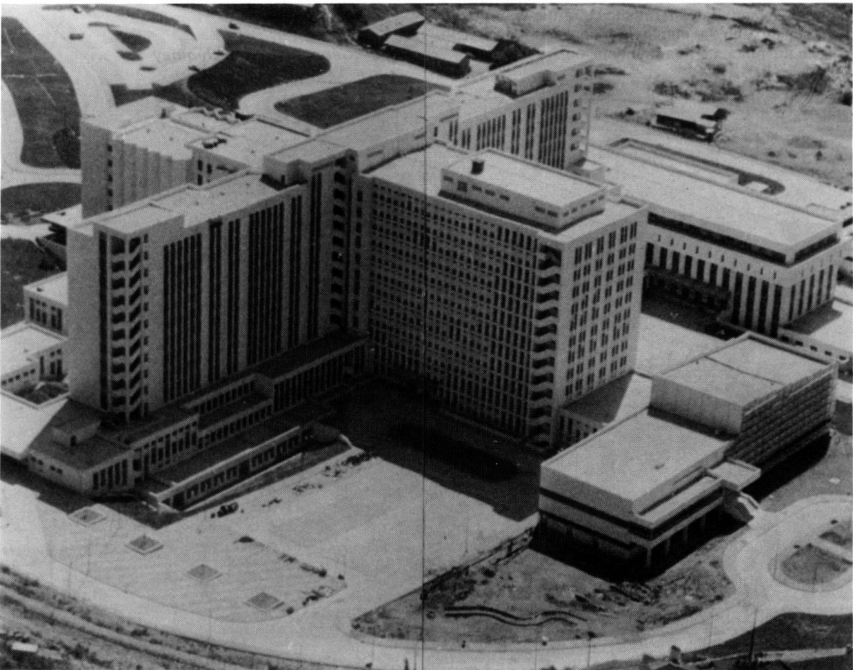
Fig. 4 View of the completed building
