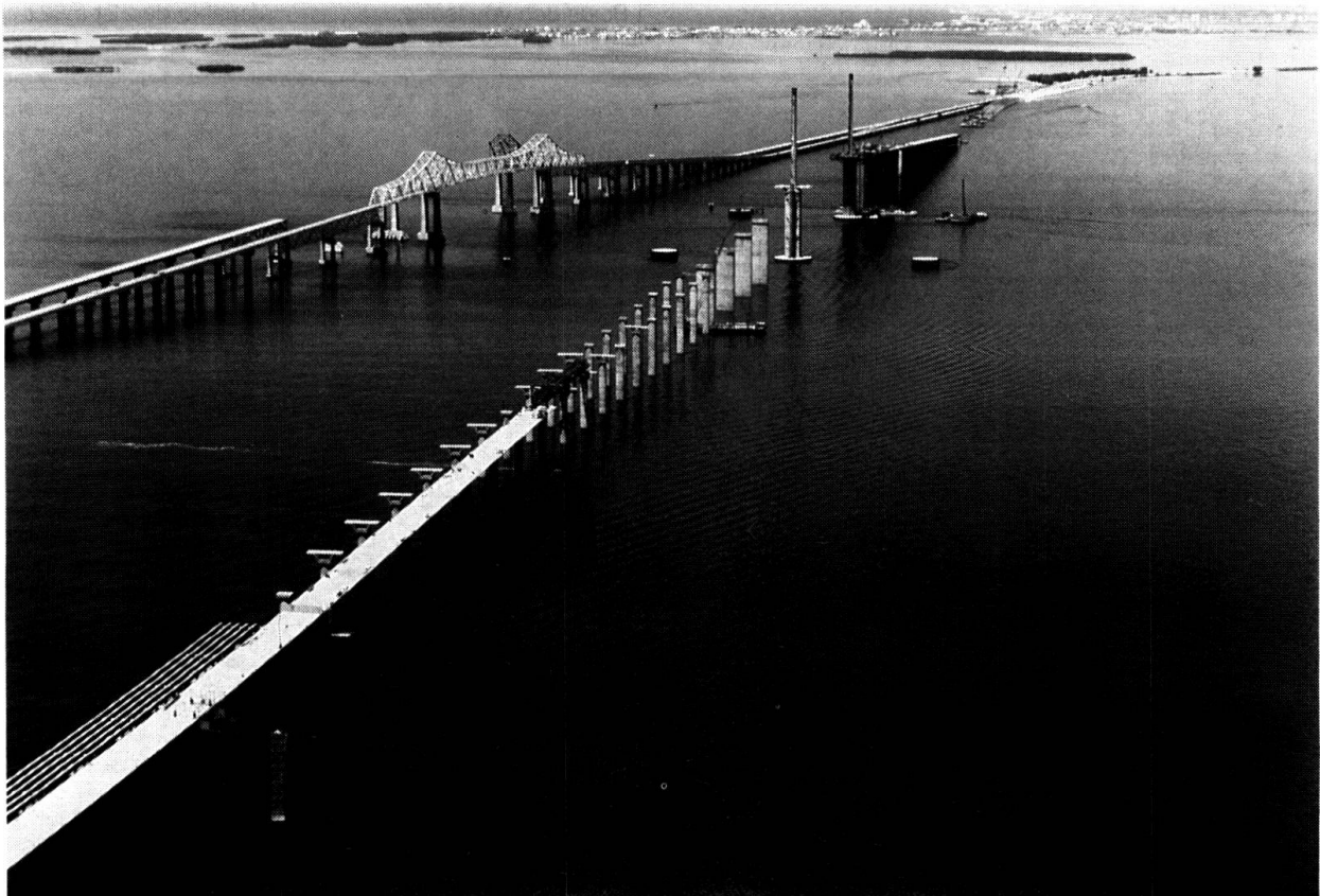
View during construction, clearly showing the various parts of the structure
