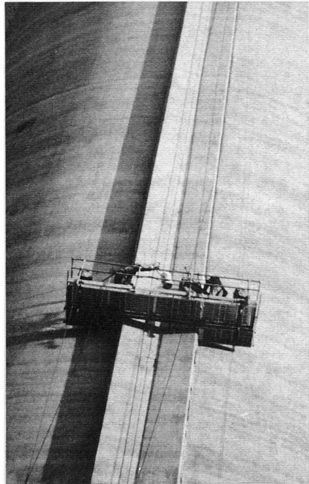
Fig. 5 VSL crew scaffold doing post-tensioning operations
