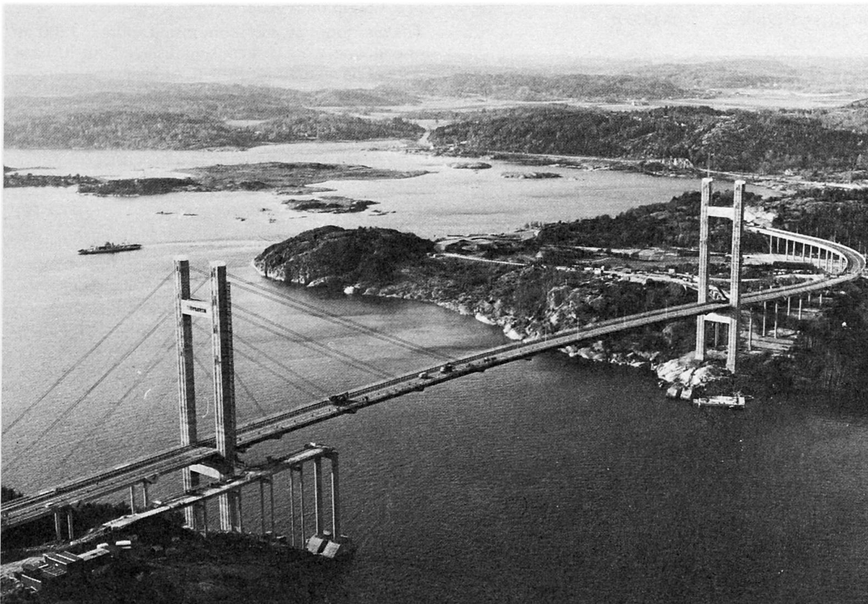
Fig. 3. The finished bridge
