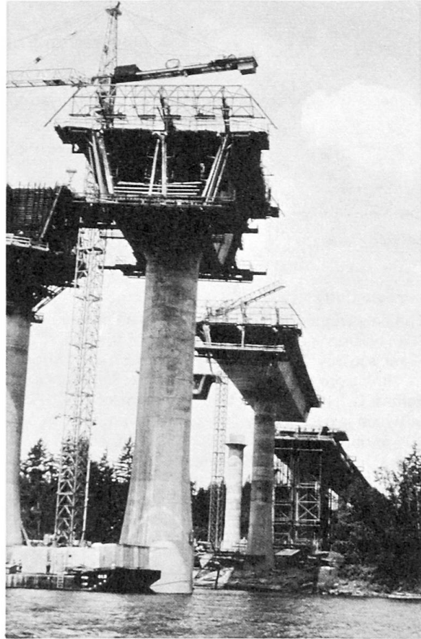
Fig. 3 Cast-in-place falsework Cast-in-place cantilever
