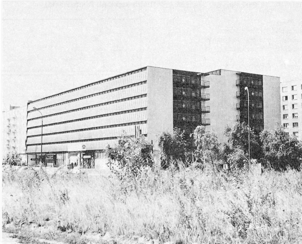
Fig. 5 Multi-garage-building at Bratislava
