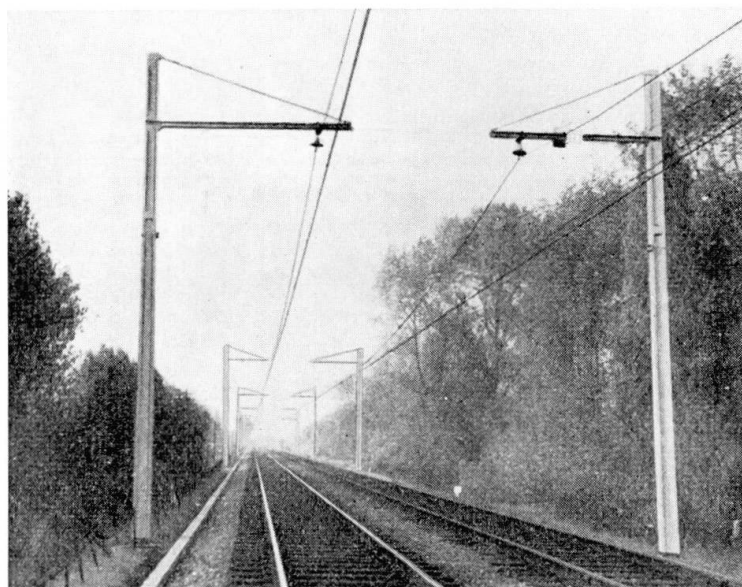
Fig. 1. Prestressed Concrete Cantilever Masts near Southend (England).
