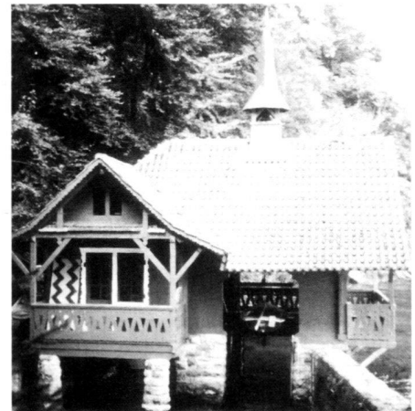
Protection of the many, valuable small buildings which make their mark along the lakeshore, such as bathhouses, pavilions, landing facilities, etc. (Horw).
