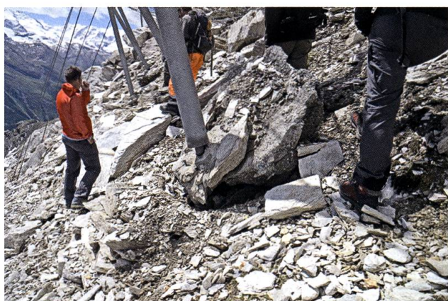
Fig. 4: Misaligned and damaged row of avalanche defense snow nets in a permafrost talus slope at Wisse Schijen (Randa, Canton Valais), resulting from differential downslope deformation and subsidence of the active layer.
