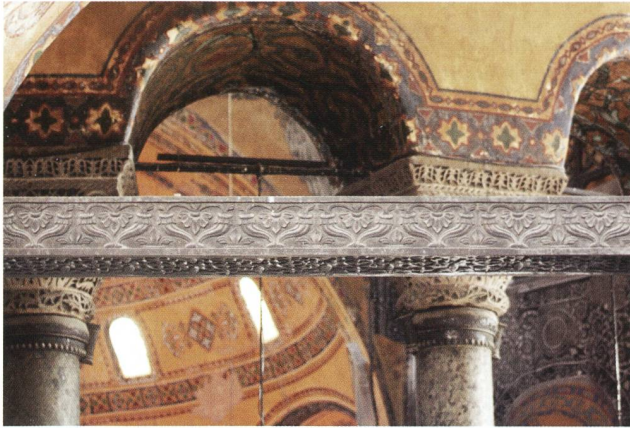
III. 6 Wooden beams replaced by Fossati, Imperial lodge, Saint Sophia, Istanbul.
