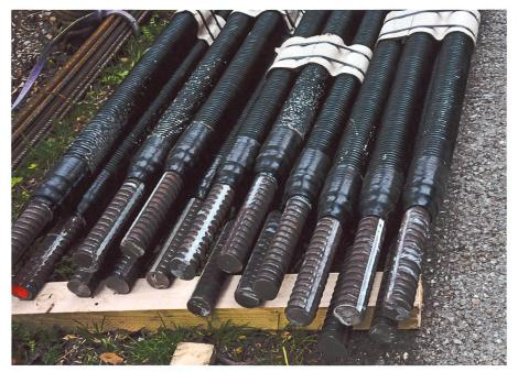
Figure 4. Ancrages type GEWI Rock Bolt.
