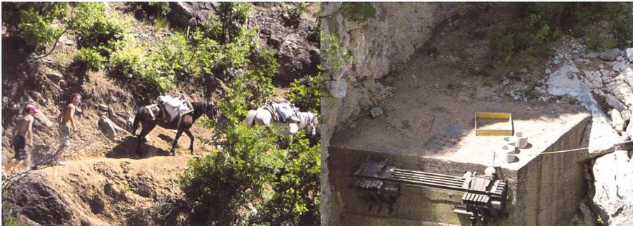
Figure 6. Transport of construction material, Mules, improvised cable cars.
