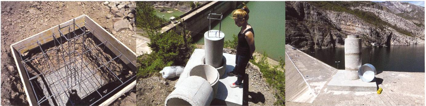
Figure 5. The construction steps of a double-wall pillar, foundation, concrete, finish.
