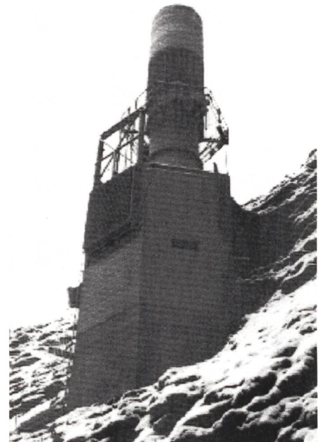
Figure 7. Prise flottante barrage Z'Mutt.
