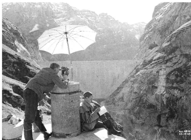
Reference number 2.130(3). Reference point with theodolite. The concrete pillar is protected to avoid thermal influences.
