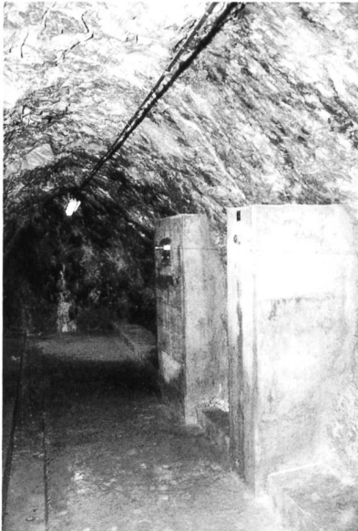
Reference number 2.110(1). Wire alignment. Measuring point in a gallery. The alignment is extended into the flanks of the valley by means of galleries to reach stable suspension points.
