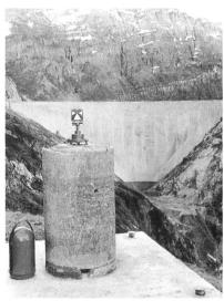
Reference number 2.130(2), above. Reference point on a concrete pillar with optical target.
