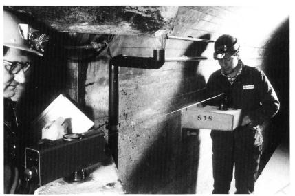
Reference number 2.111. Levelling inside a concrete dam. In the rear the levelling instrument on a tripode; in front the target scale is illuminated by an electric torch.
