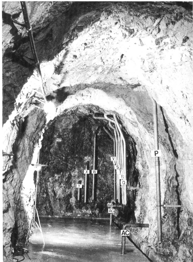
Reference number 2.200(1). Drainage gallery with pipes collecting seepage water. The seepage can be measured with a calibrated container and a watch for each pipe separately. (Photo Feuerstein)
