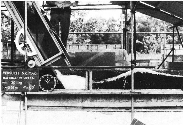
Figure 3. Impulse wave generation by a plunging ice mass in a two-dimensional model.
