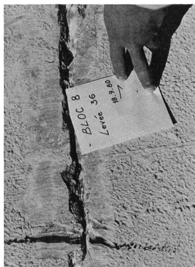
Figure 8. Crack to be sealed before injection.
