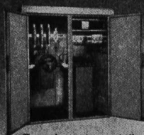
Transformatorstation in Freiluftkabine 50 kVA, 1000/220 V
