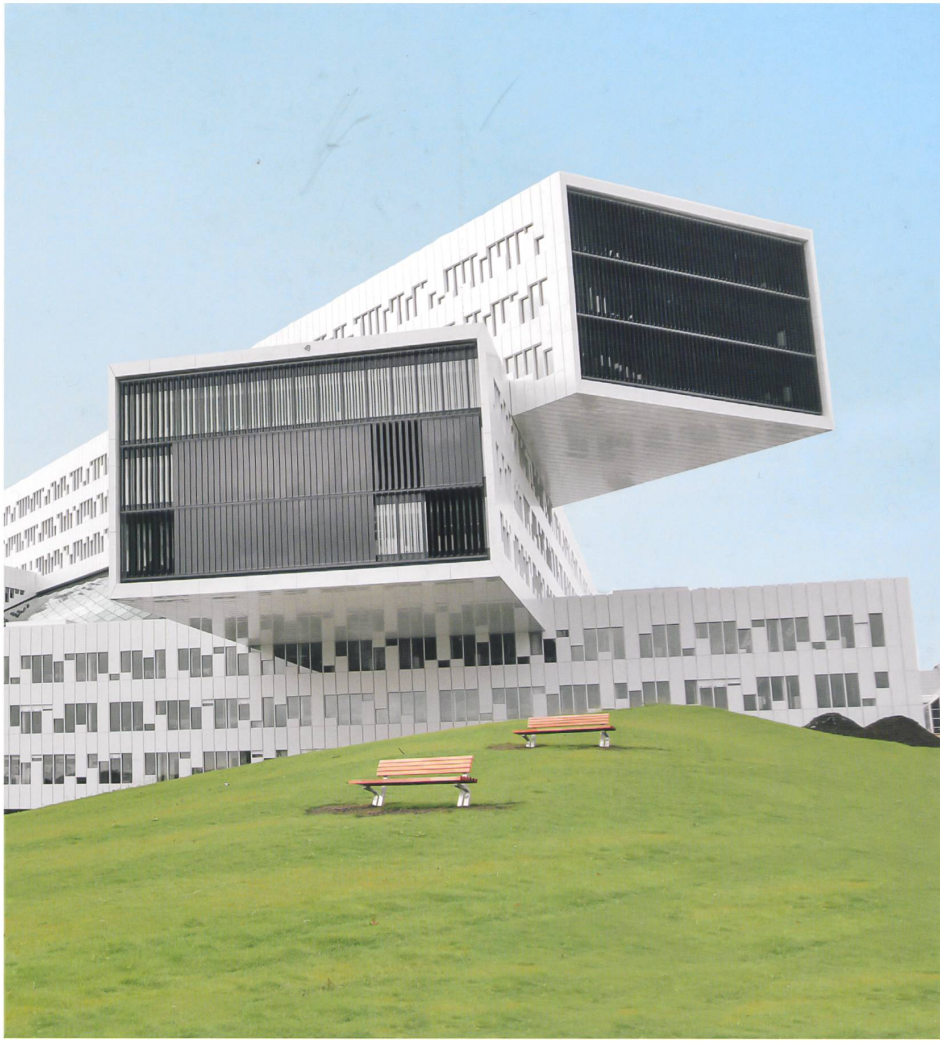
Statoil Headquarters, Oslo
