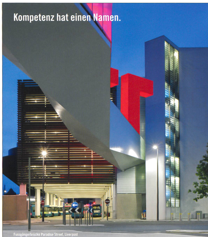
Fussgängerbrücke Paradise Street, Liverpool
