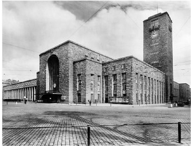
Hauptbahnhof in Stuttgart, 1911–27
