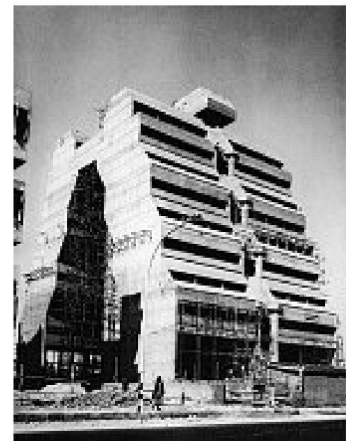
NCDC National Cooperative Development Corporation Office Building, New Delhi 1974–78, Mahendra Raj mit Kuldip Singh.
