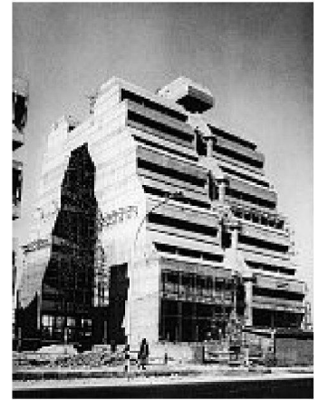
NCDC National Cooperative Development Corporation Office Building, New Delhi 1974–78, Mahendra Raj mit Kuldip Singh.
