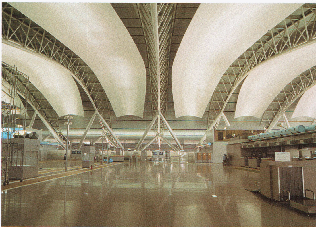
Haupthalle Hall principal Main hall
