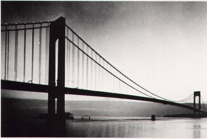
Verrazano-Narrows-Bridge, New York 1964
