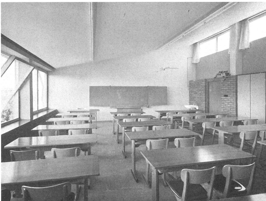
Klassenzimmer Hauptbau, 2. Stock | Salle de classe; bâtiment central | Classroom of main building, 2nd floor
