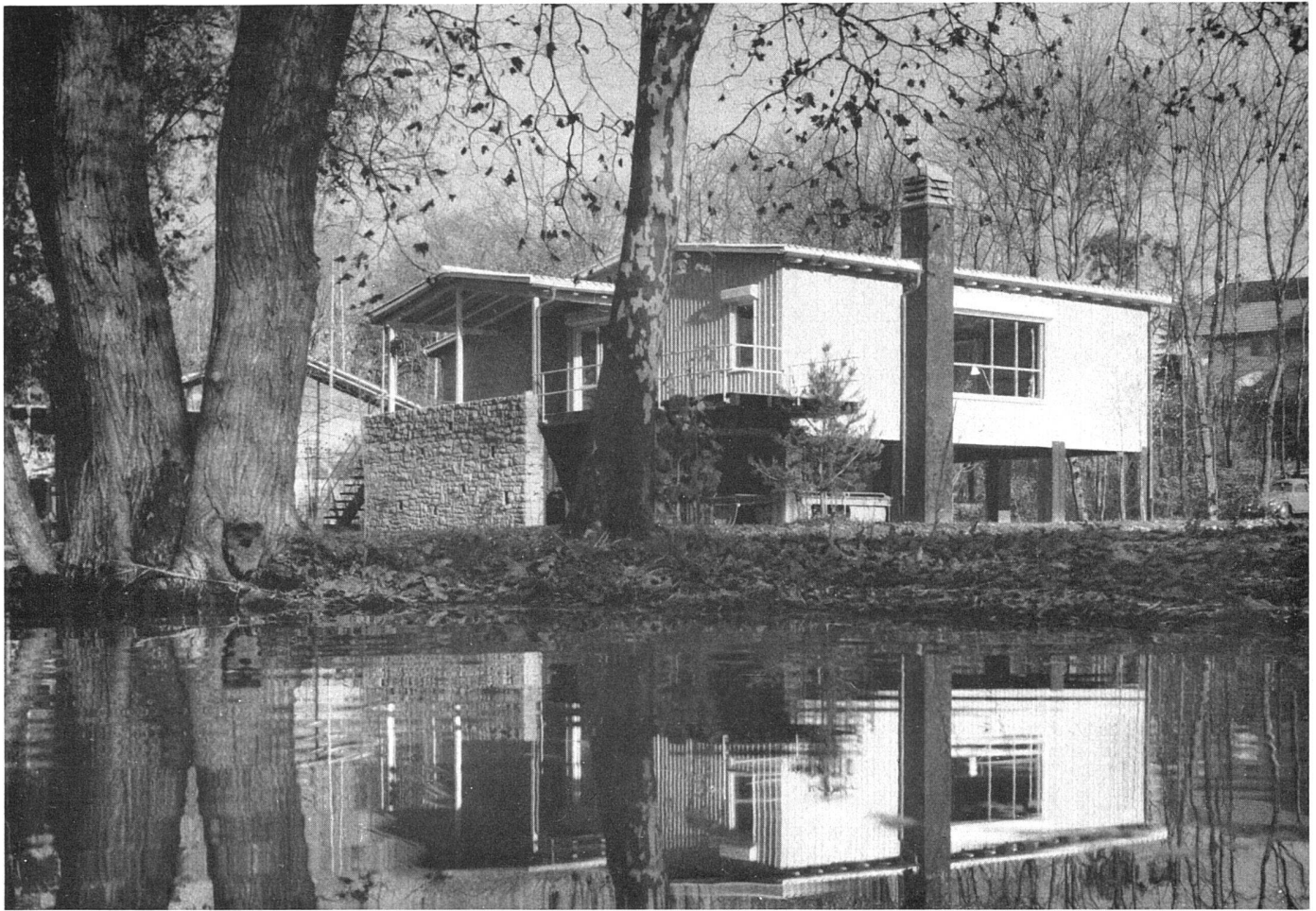
Gesamtansicht vom See | Vue prise du sud-est | Water front from the south-east
