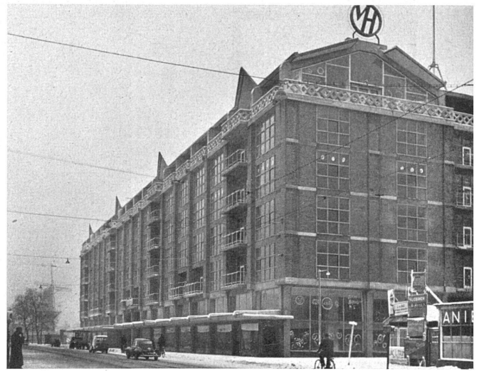
Mietfabrik Goudse Singel. Ladenfront | Usine locative (II), vue générale | General view of flatted factory (II)
